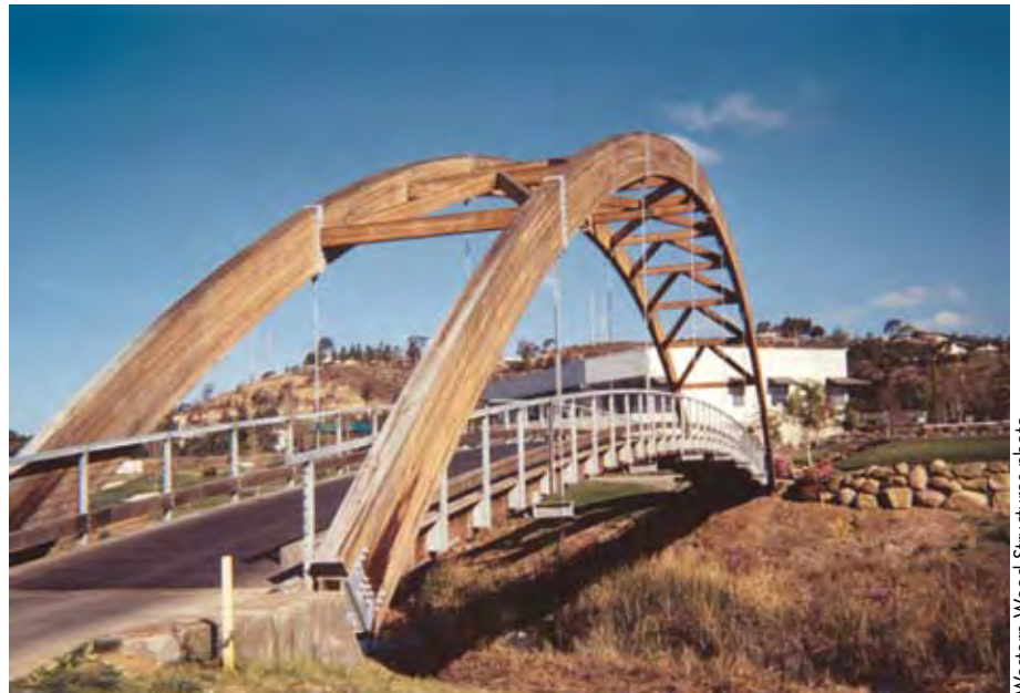
Glulam bridges spanning 117 feet and 170 feet provide graceful crossings at the Riverwalk Golf Club.
