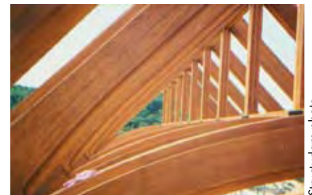
Mt. Fuji Golf Club in Chiba, Japan, uses glulam trusses with very intricate detailing, designed to look like furniture.
