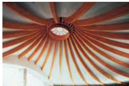
Radial glulam arches in the 21st Century Golf Club in Takasaki-Cho Gunma, Japan, provide a good example of the design versatility of glulam.
