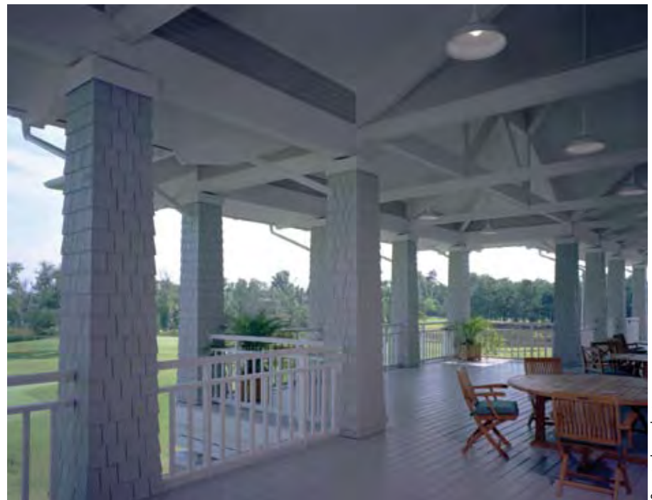
Glulam trusses complemented the comfortable environment of the Eagle Point Clubhouse.
