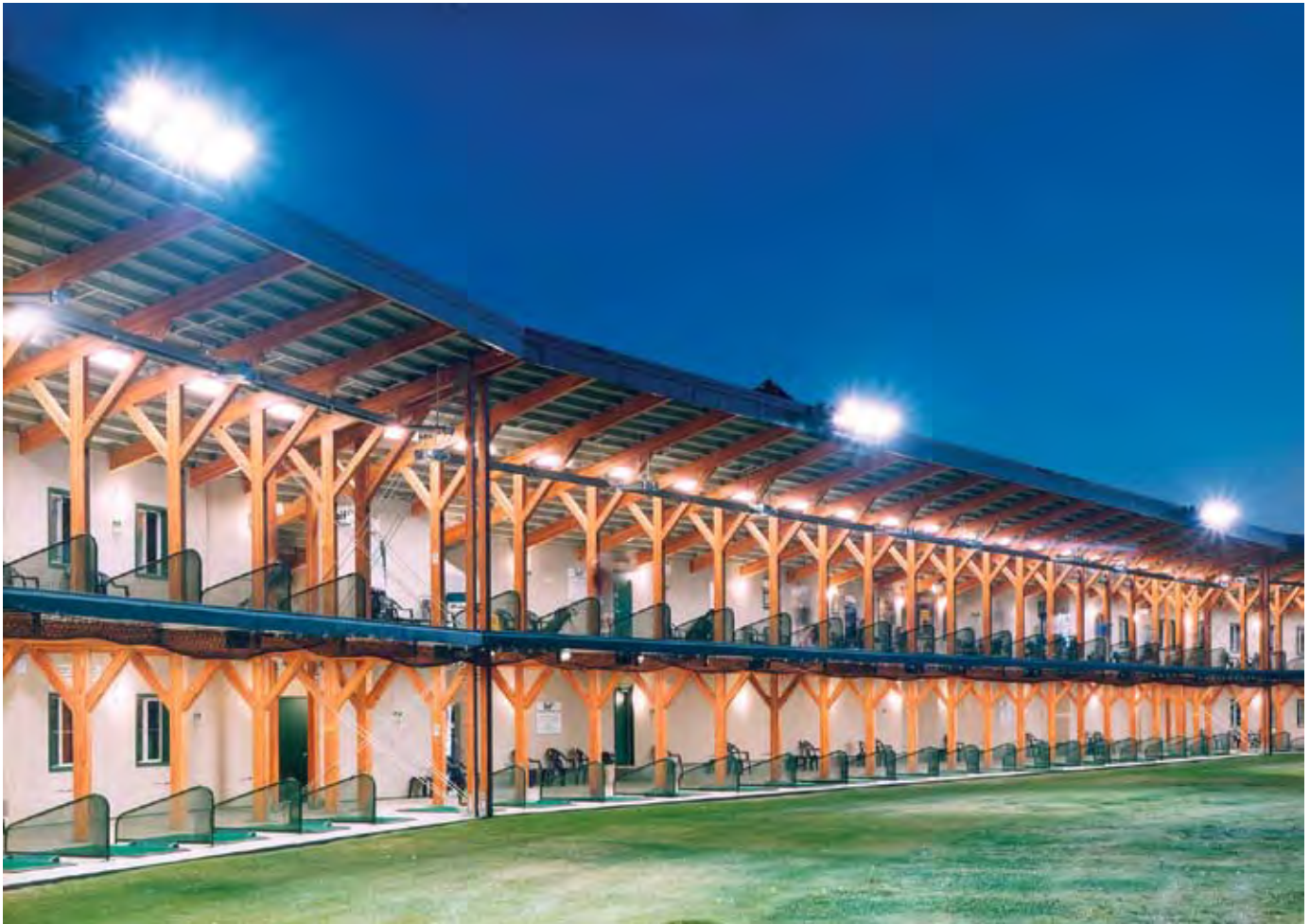
By having their driving range structure re-engineered, owners saved money by better utilizing wood's natural compression strength and eliminating many of the steel connectors.
