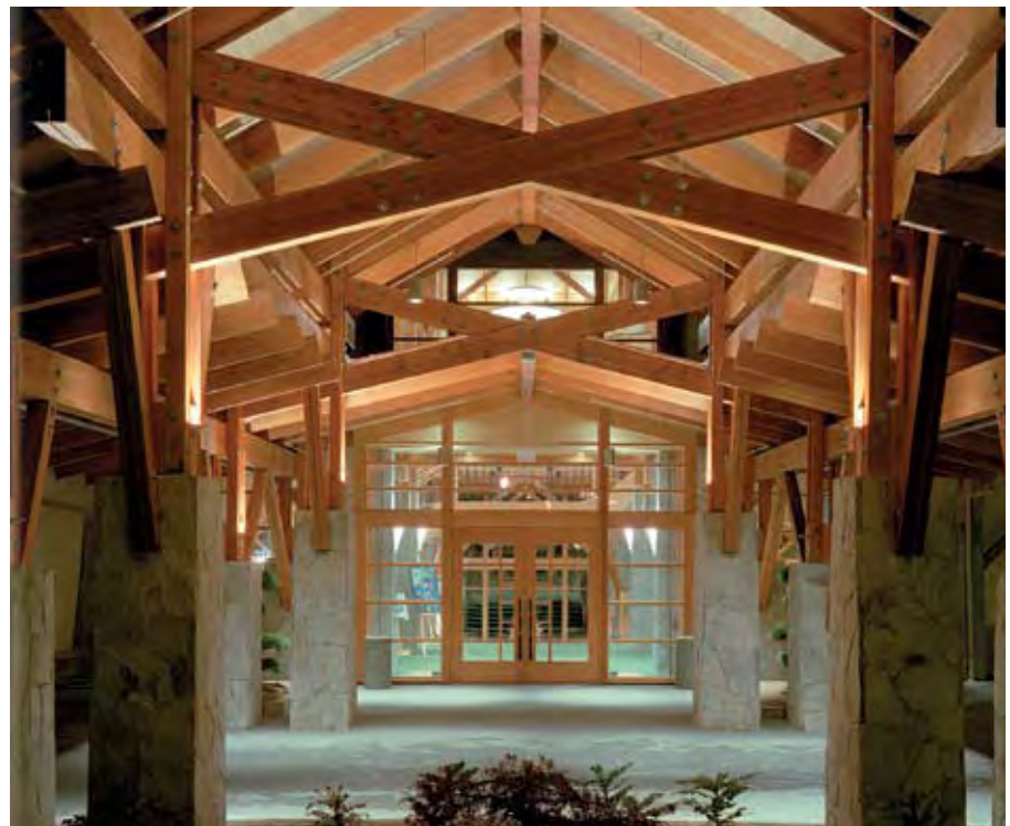
Westwood Plateau’s architects wanted to design a project with high level of structural expression, so they developed a glulam system that allowed the building to frame itself in both directions with cross-bracing elements.
