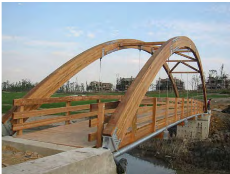
Western Wood Structures photo
