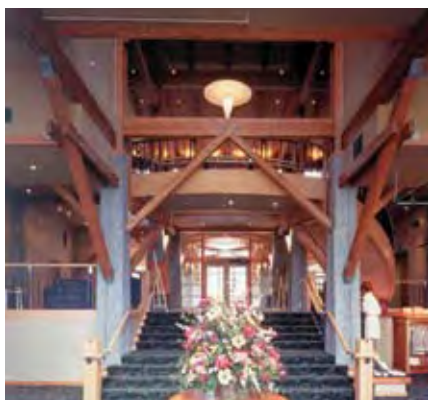
Structurlam, the glulam fabricator, used a wire brush to give these beams an interesting, rustic finish. The process made them look like solid timber, yet the beams still provided the structural performance of glulam.
